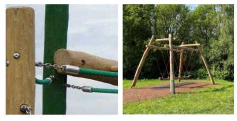
Above: Broadstone Recreation ground, high quality rope and rope fixings, a wear pad installed under the new rope, swing will ensure long term, durability of the surfacing in a high friction zone.
